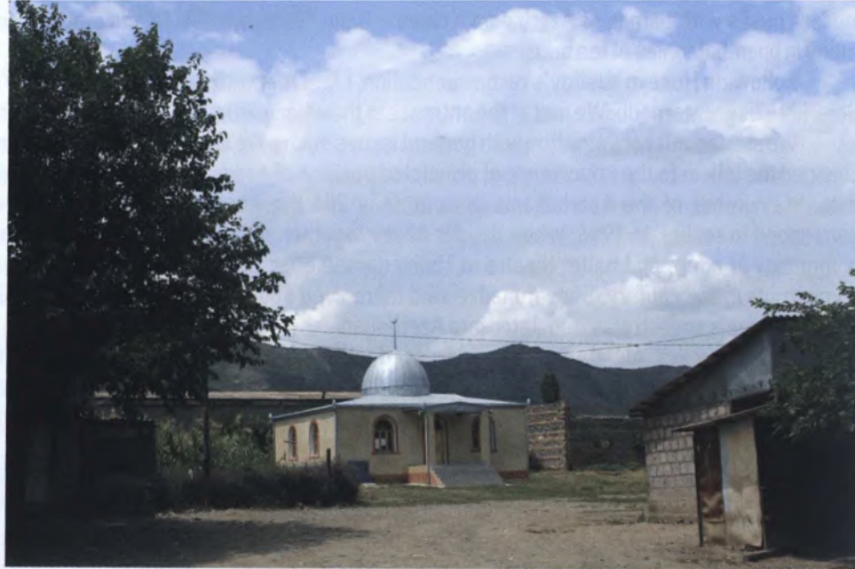
New mosque of Demye Gorarkhi village
