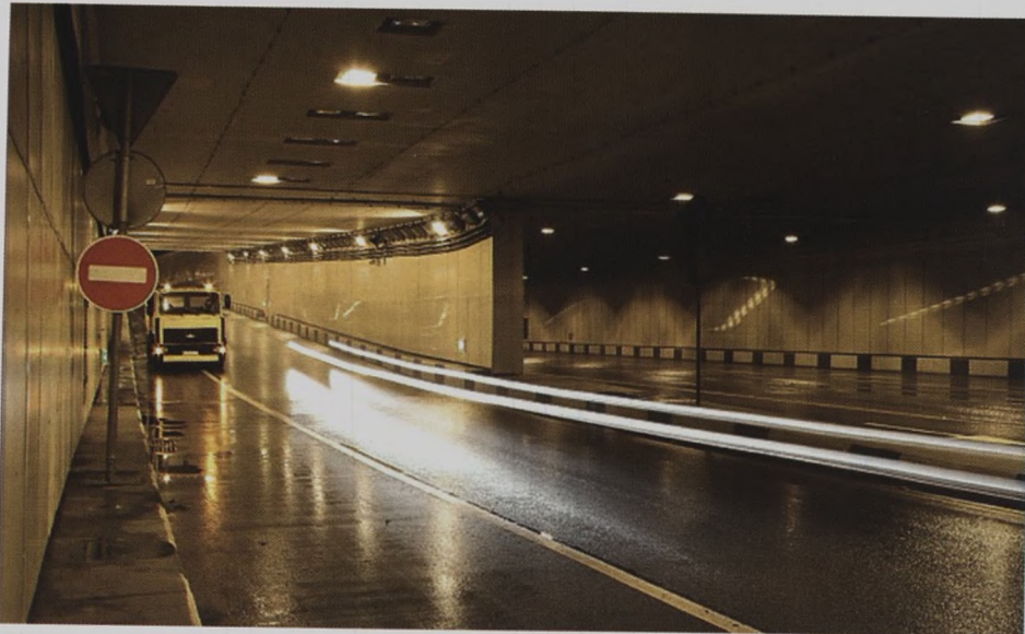
Lefortovo avtomobil yolu tuneli (RF).
