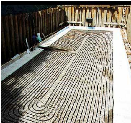
Figure 2. Laying pipes under the foundation slab
